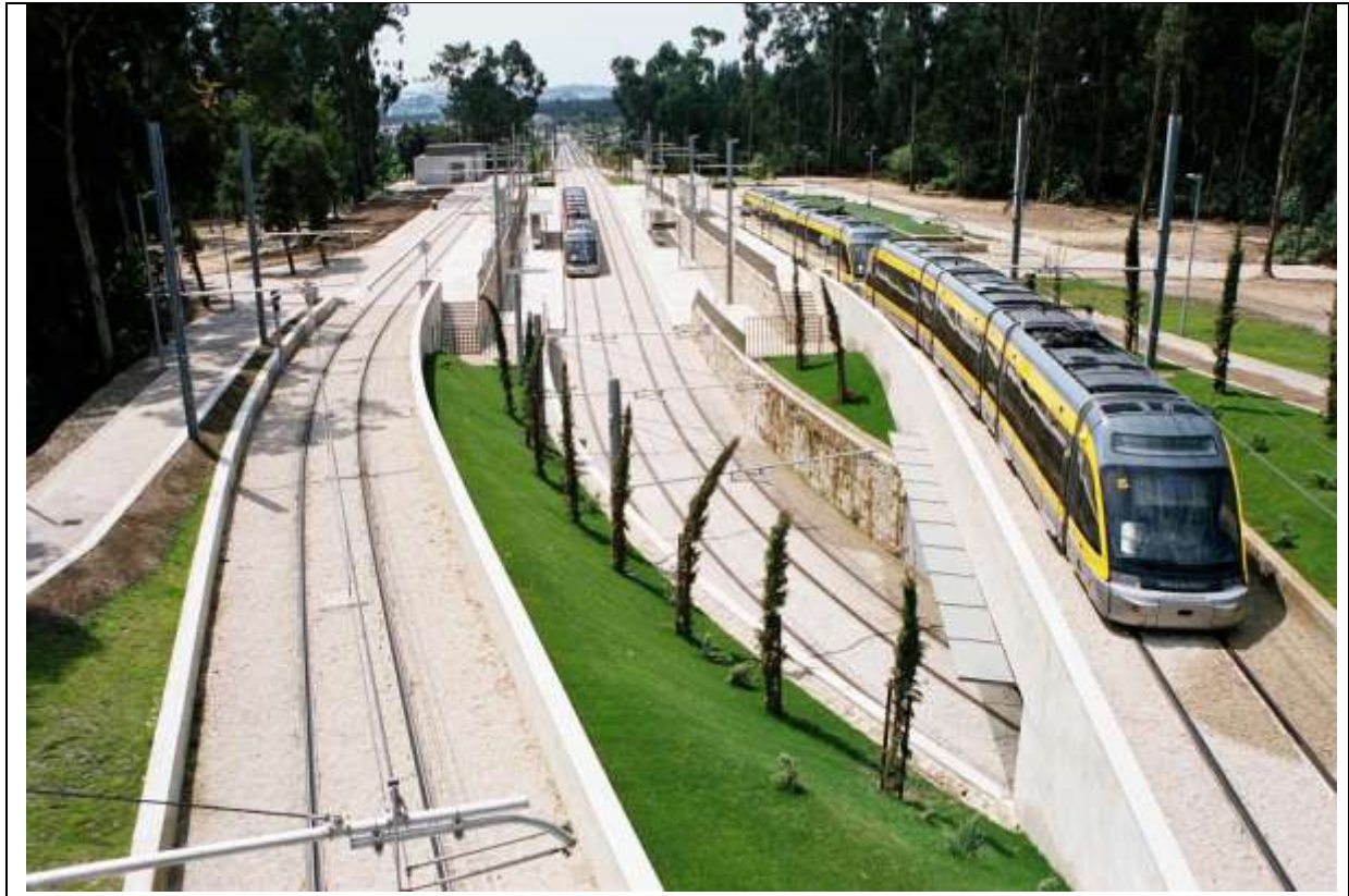
Figure 32 – Porto grade separated light rail junction
