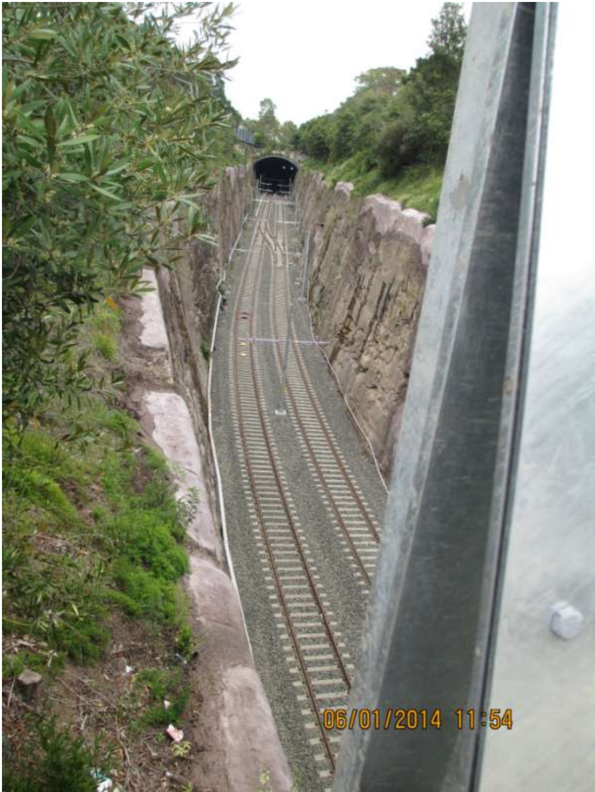
Figure 14 – View of current Inner West Extension west of Lilyfield showing Overhead Support Poles in the Rock Cutting
