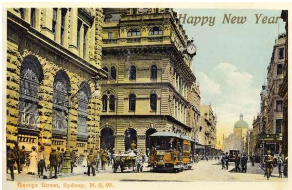
Figure 7 - George Street c1909 at Martin Place (note Centre Poles have been removed, much of the overhead is now supported directly off buildings to minimise the number of street poles)
