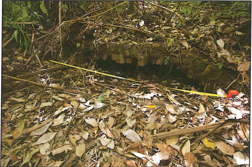
Photos of historic cistern structure which will be impacted on by the proposed development
