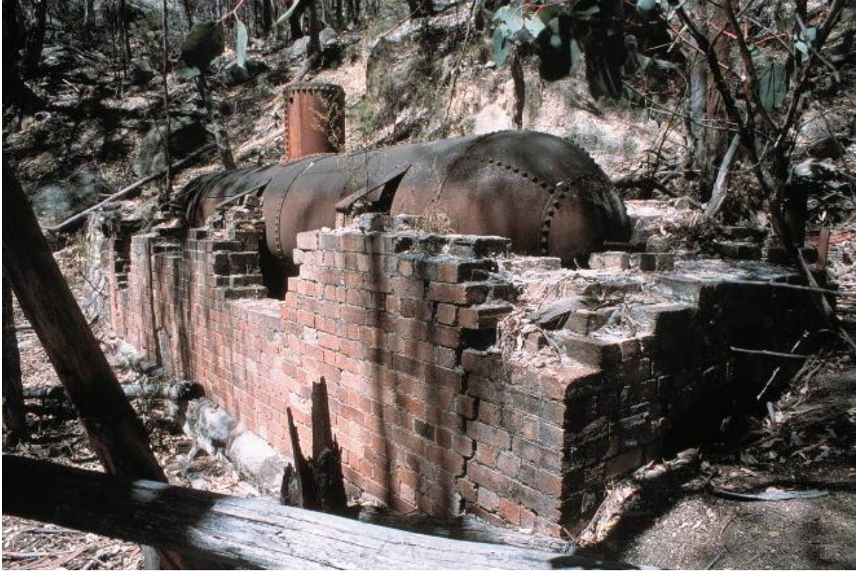
Figure 8: Egg-end boiler associated with the Cable tramway haulage system (Source: Ayling, B op cit)
