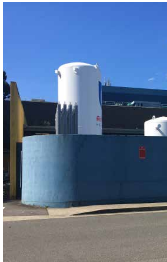
Fig 27: View of bulk oxygen supply
