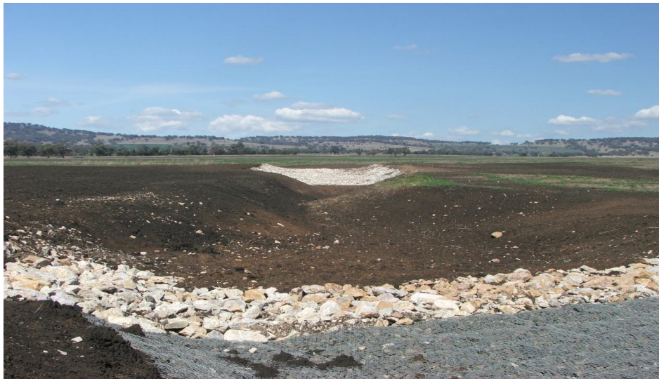
Photo 3: Looking uphill along rehabilitated pipe crossing failure at gully at “Barana”
