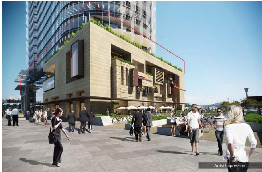
Figure 13 Required increase in height to the podium as shown in red to address wind wash
