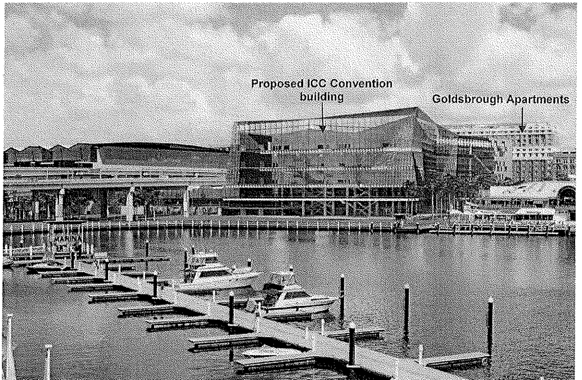
Photo 7: View of the proposed ICC Convention from eastern foreshore of Cockle Bay (source: SICEEP SSD report)
