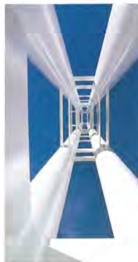
Tubular steel masts support the roof over each hall. Photo: David Moore.
