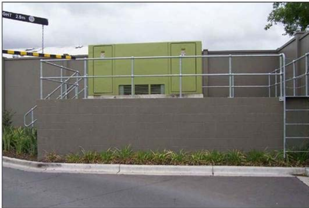
Figure 51 - Example substation raised above 1:100 flood level
