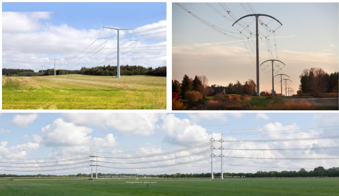
Figure 13 - Hinkley Connection Project 400 kV double-circuit (top left), BOLD Transmission 345 kV double-circuit (top right) and two 380 kV double-circuit Wintrack lines
