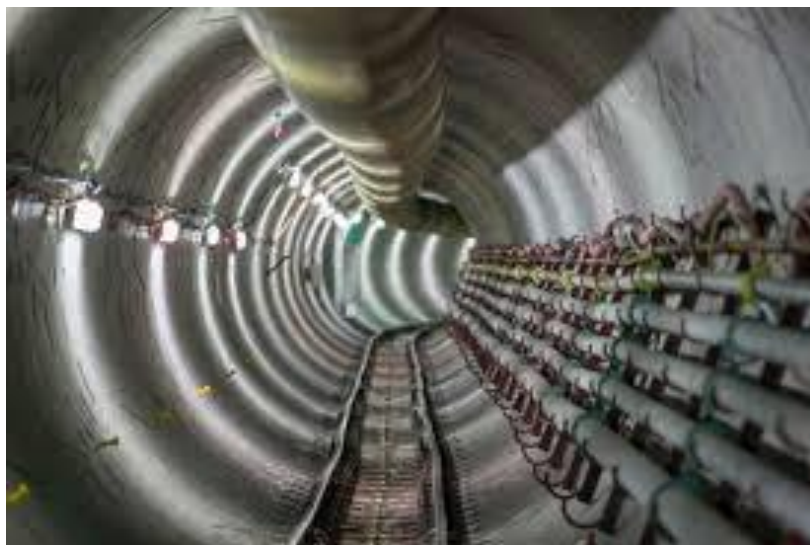
Figure 8 – Sydney City East Cable Tunnel (3.5m diameter) 55
