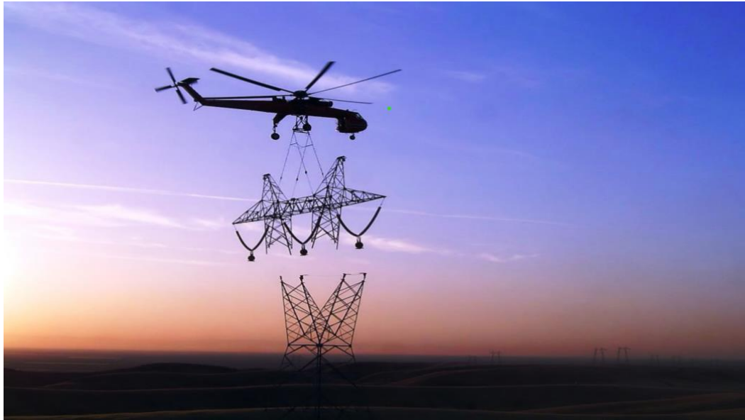
Figure 14 - Helicopter Construction BPA McNary-John Day 500 kV Transmission Project
