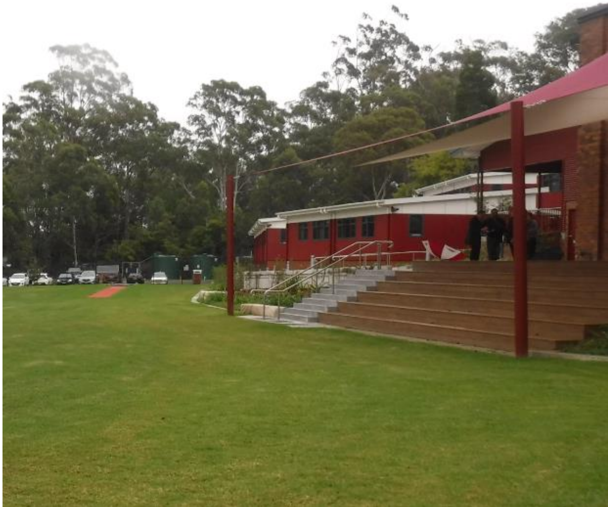
Figure 4.6: Existing Raised Building at Envelope 5
