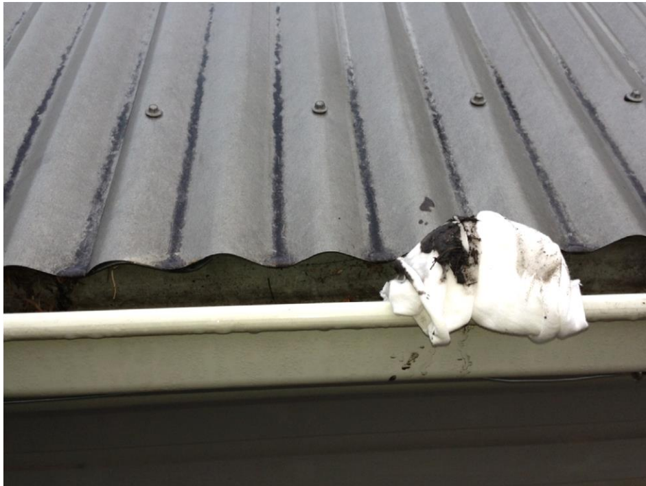
Black dust at 20 Yarraman Rd in roof corrugation valleys. The rag was lightly wiped in the guttering. This is the collection path for our drinking and house water
