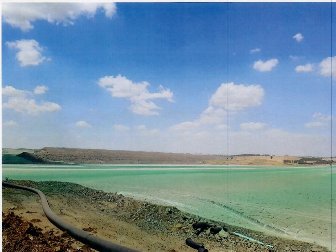
Figure 5. 3/1/2020 STSF looking back towards the NTSF wall (slump on the left) the day after aerial campaign suspended
