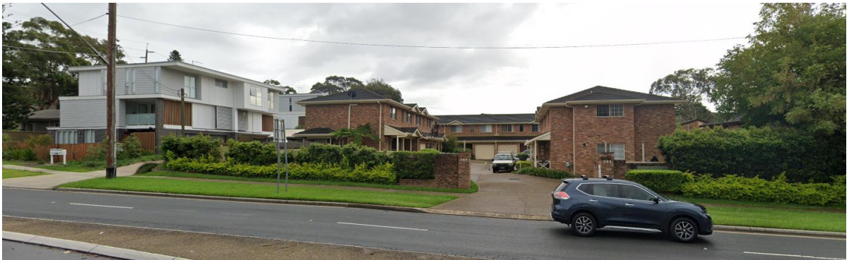
Figure 3: Street elevation of President Avenue east of President Private Hospital looking north showing mix of two and three storey residential buildings
