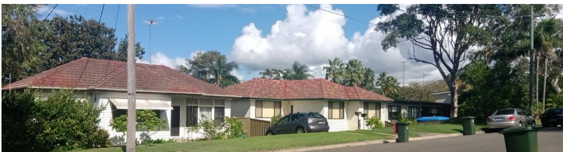
Figure 9: Street photos of 4 and 6 Bidurgal Ave. No 4 is to be demolished for the redevelopment No 6 will be adjacent to the new north wing. No 2 (not shown) is a two-storey brick house to be demolished.
