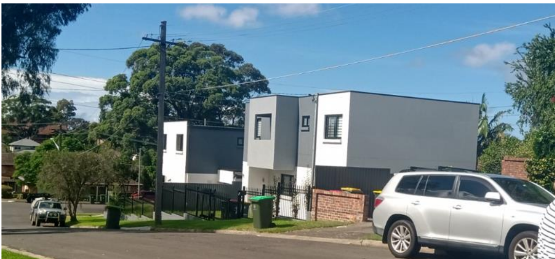
Figure 8: Street photo looking east along Bidurgal Ave showing the duplex at No 59 Hotham Rd
