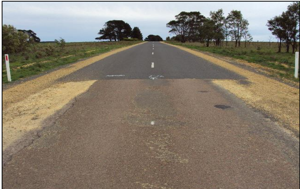
Figure 5.2: Typical unsealed increase in width of (public) road
