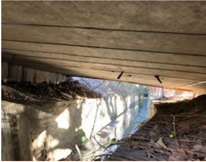
Figure 5. Concrete plan bridge decking (underside) spanning concrete lined canal approx. 100m north of the buildings. Water was present in the canal during the diurnal survey.
