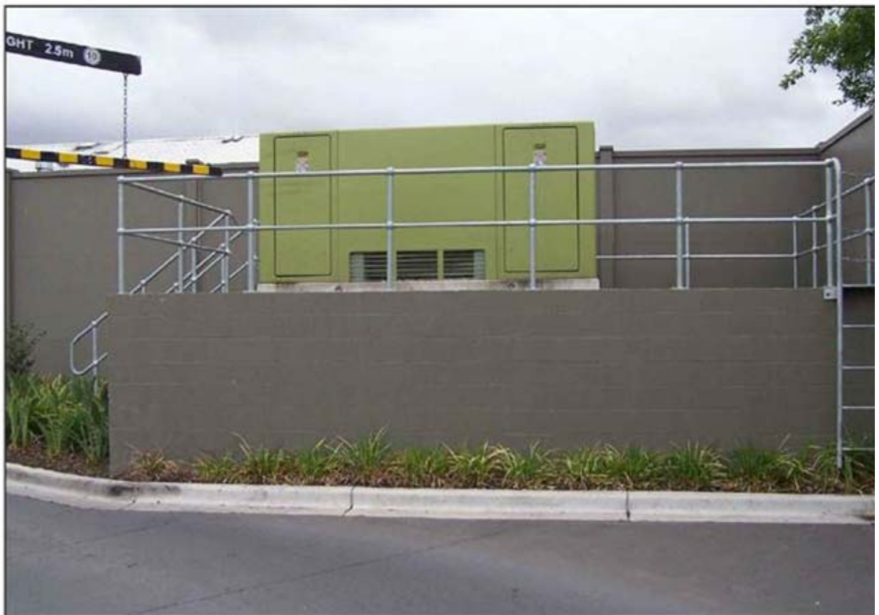
Figure 51 - Example substation raised above 1:100 flood level
