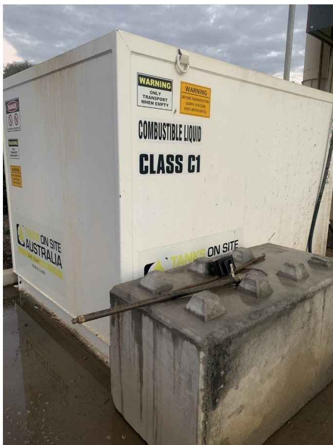
Photo 27: Double skinned / bunded diesel fuel tank.
