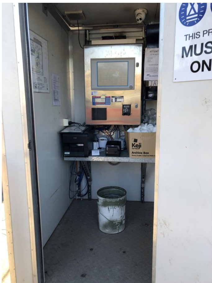
Photo 24: Waste logging and sampling point to be undertaken by the driver of the delivery vehicle. The machine logs the sample with the respective provider, including company ID, driver ID, vehicle registration and waste description.
