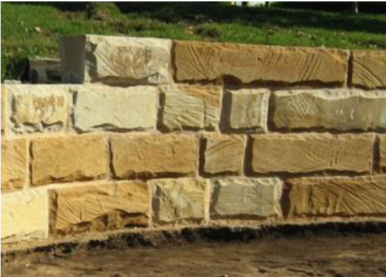
SANDSTONE RETAINING WALLS
