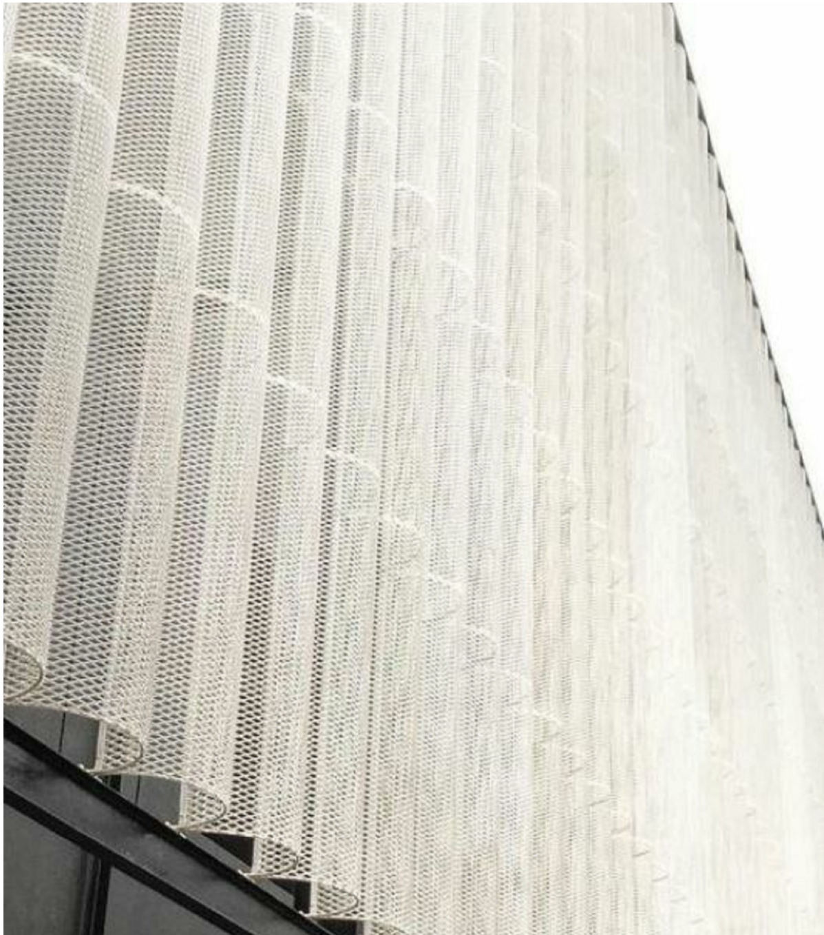
1. PERFORATED SCREEN - ALUMINIUM, FINISH - POWDERCOATED WHITE
