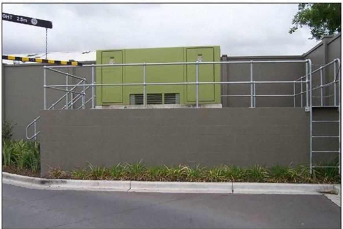
Figure 51 - Example substation raised above 1:100 flood level
