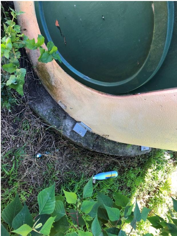
**Figure 2-7 Exterior of bus shelter showing attachment to concrete pad, and revealing orange colour beneath green paint**
