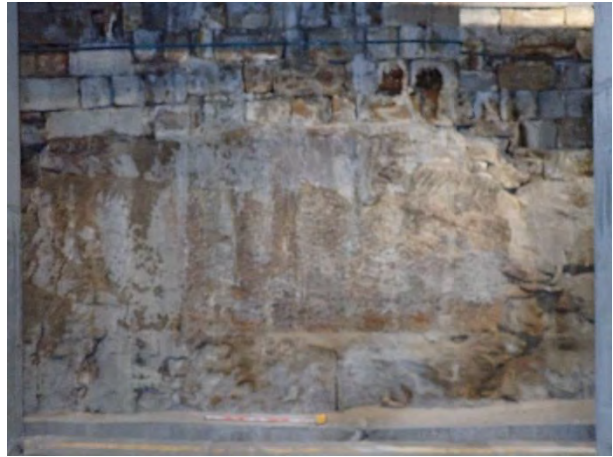
Figure 49 – sandstone bedrock cut for the boiler room basement, with sandstone blocks present on top of the bedrock.
