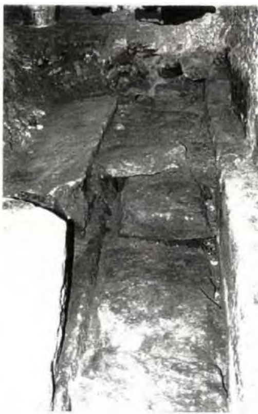
Figure 24 – Box drain associated with south wall of Cleland Bond Store, Johnson 1996.
