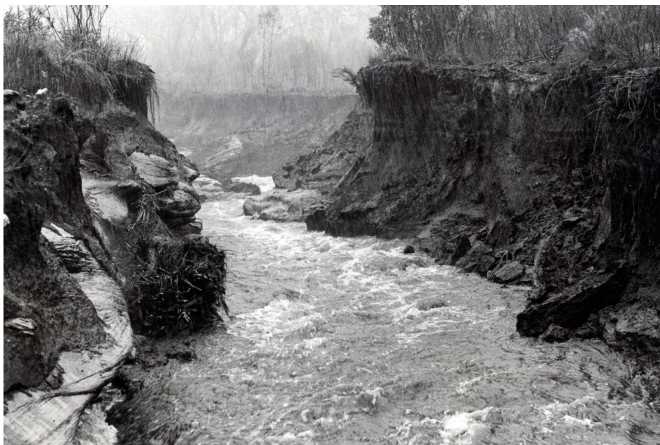
Drillhole Swamp did not collapse due to exploration drilling or bushfire, it collapsed due to tilting of the underlying rock strata. Photo: A. Young
