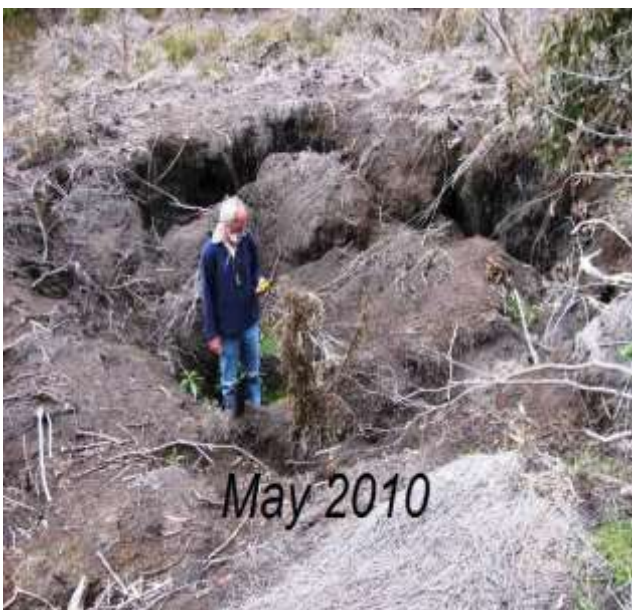
Photo 17: Sinkhole East Wolgan Swamp on 16 May 2010
