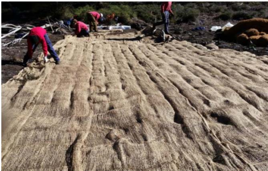
Figure 3 - Slumping Area in Figure 2 in Process of Rehabilitation in Accordance with Section 95 Approved Remediation Plan (June 2014)
