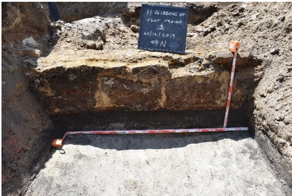
Figure 19: Exposed west face of footings exposed during test excavation at 11 Gibbons Street. Artefact 2019
