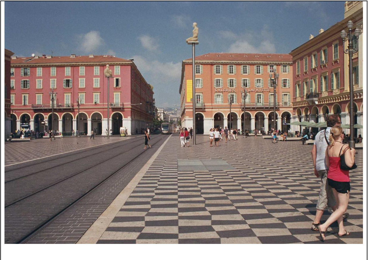
Figure 3 Nice, France Wire Free Area (note absence of APS third rail)
