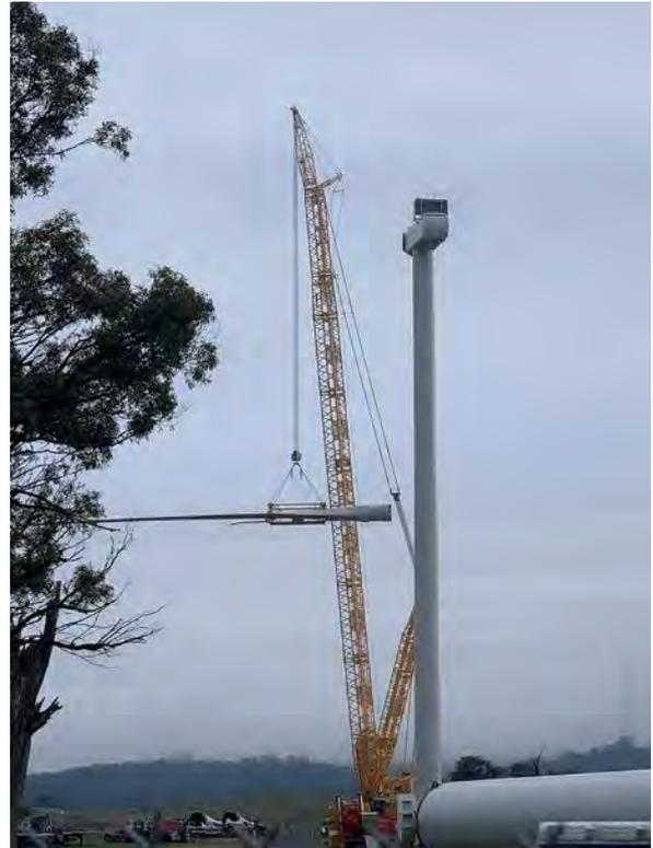
4. A view of the blades being attached to the turbine hub. Note the area needed for material laydown and construction vehicle, such as the crane, and parking (photo source: Vestas, Collector Wind Farm, NSW).
