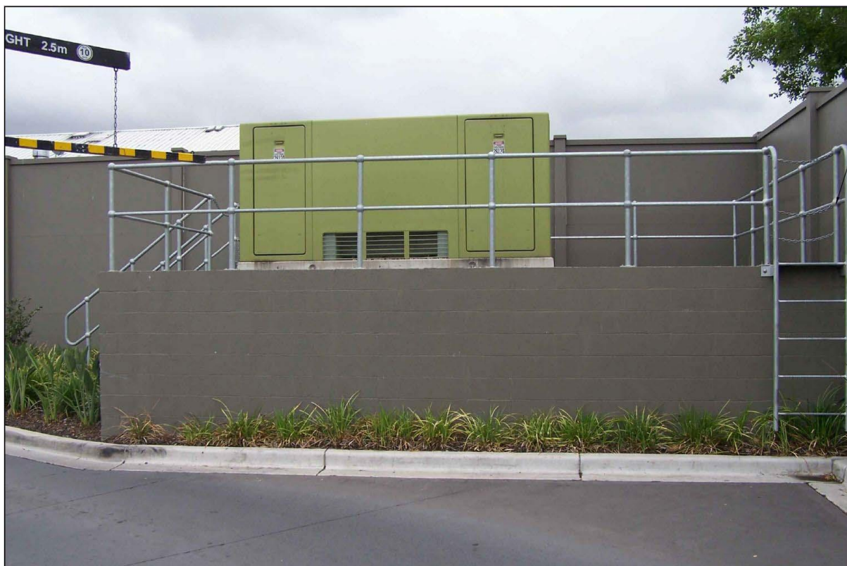
Figure 51 - Example substation raised above 1:100 flood level
