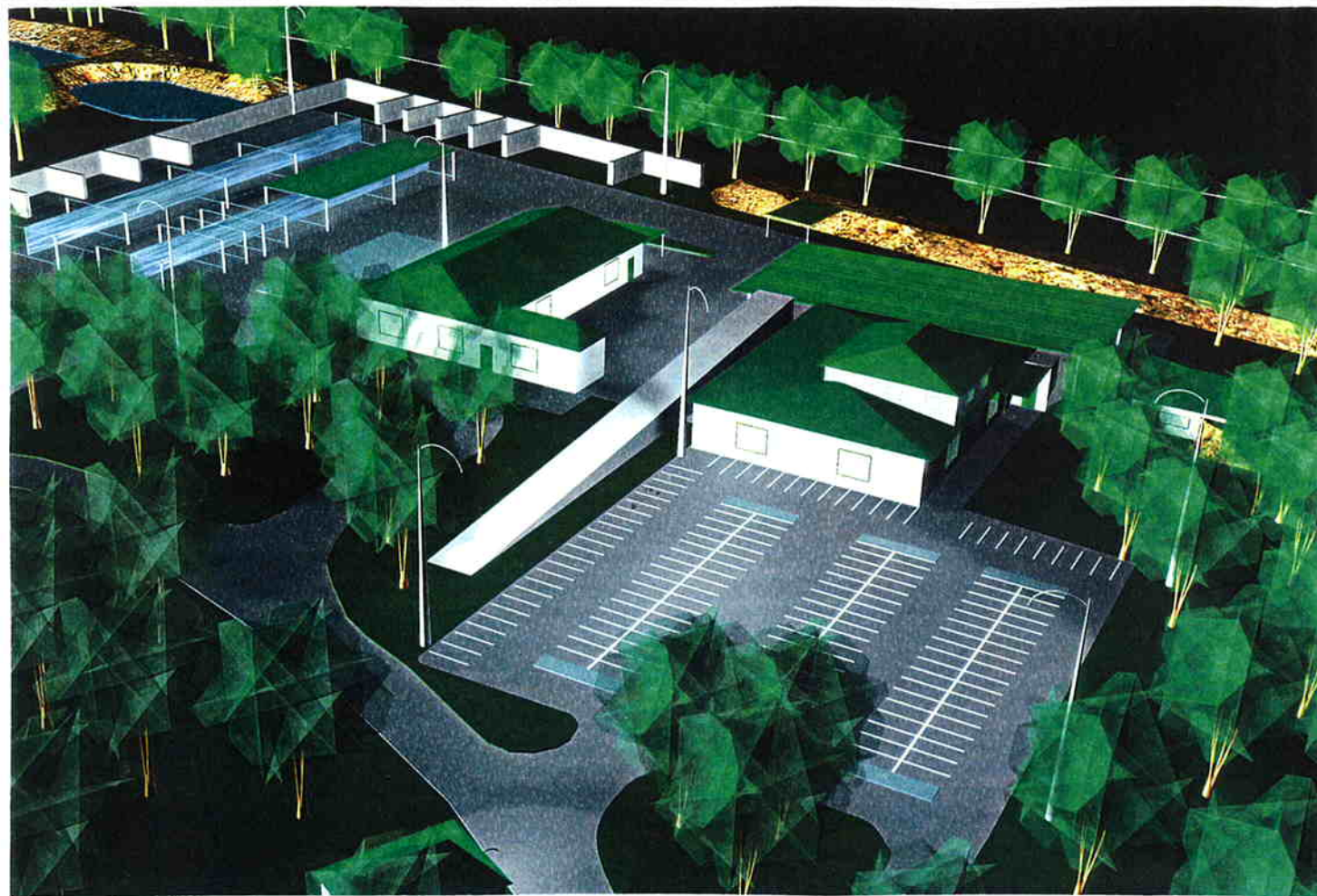
SITE ENTRY VIEW
