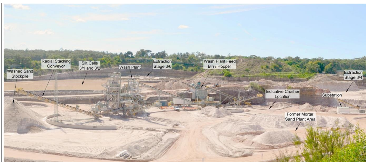
Plate 1 Processing and Stockpiling Area – Calga Sand Quarry
