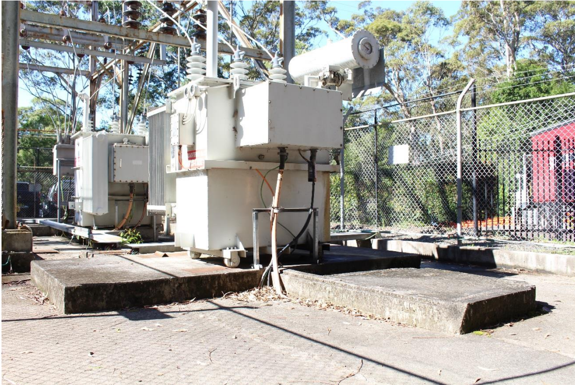
018 View of modern 33/6.6kV 1.5MVA power transformer (D-SS03-TX01) looking east south east
