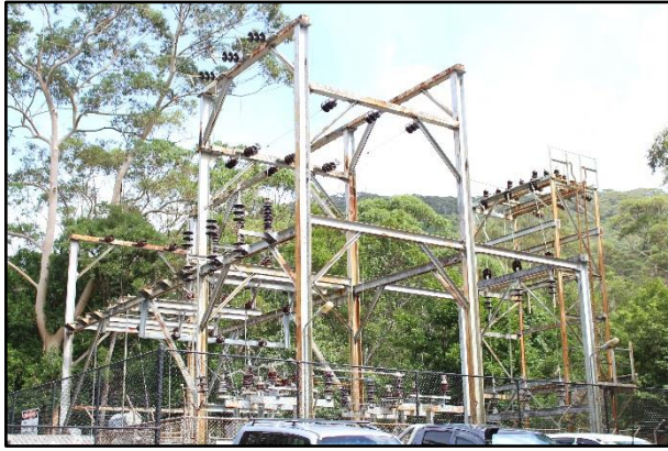
Plate 8: 3 m by 15 m steel tower with a smaller 4 m by 4m north eastern tower, south east aspect. (Source: Niche 2018).
