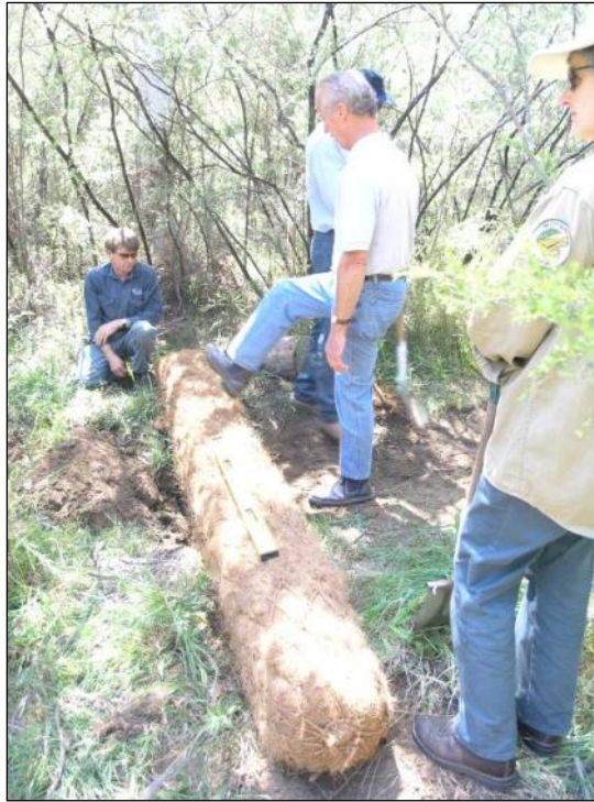
Figure 6-6 Round Coir Logs Installed to Spread Water
