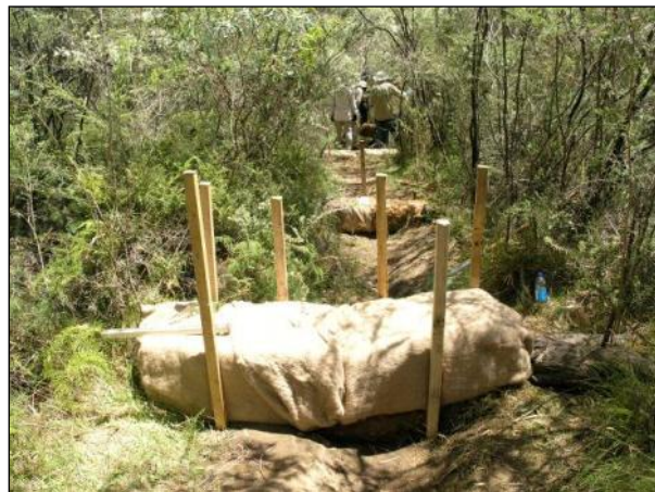
Figure 6-5 Small Coir Log Dams with Fibre Matting
