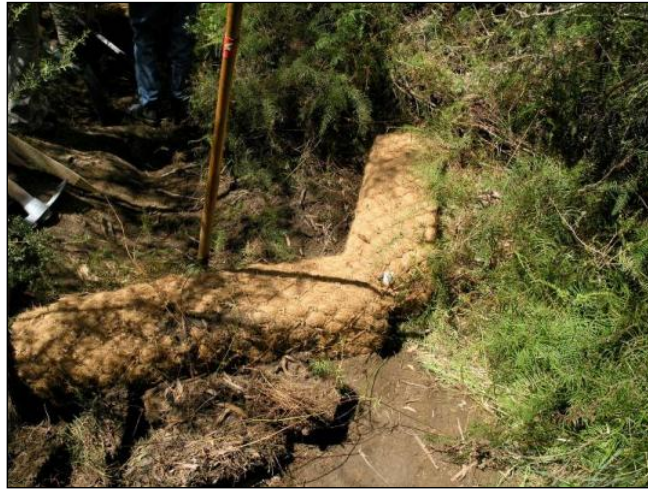
Figure 6-2 Square Coir Logs For Knick Point Control
