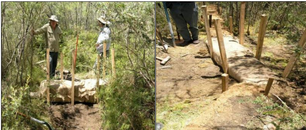
Figure 6-3 Installation of Square Coir Logs
