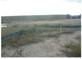
Plate 16 Silt fencing to the south of the dam construction. View to the north
