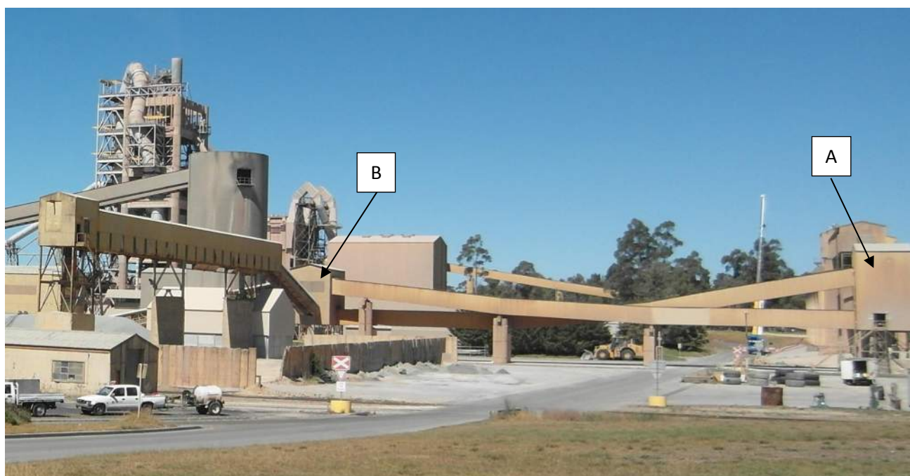
Figure 8: Location of two transfer point sources included in the dispersion model (with the emission from these two sources representing the emissions from all transfer points).
