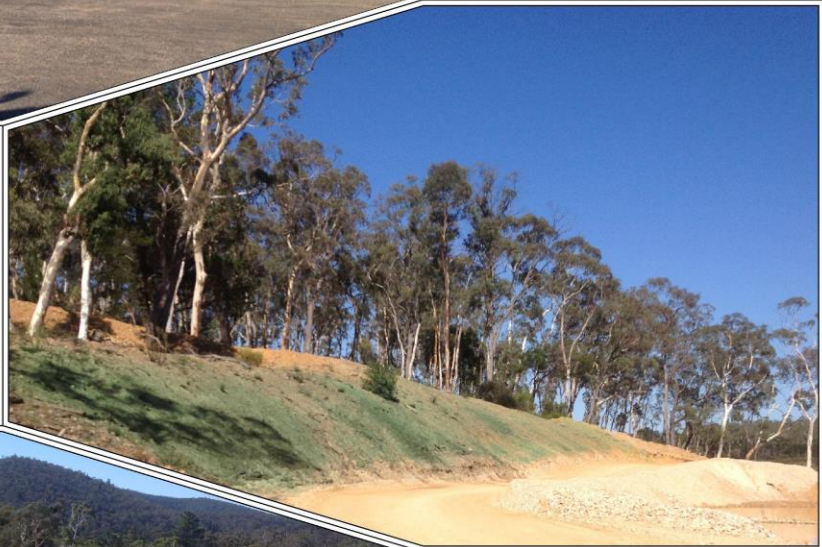
Plate 2: Hydroseeded batter above Silt Cells (Ref: IMG_3572)
