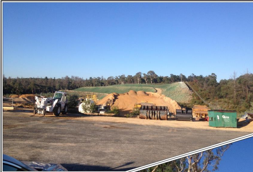
Plate 1: View of Hydroseeded batters of the Western Stockpile Area and Amenity Bund (Ref: IMG_3565)
