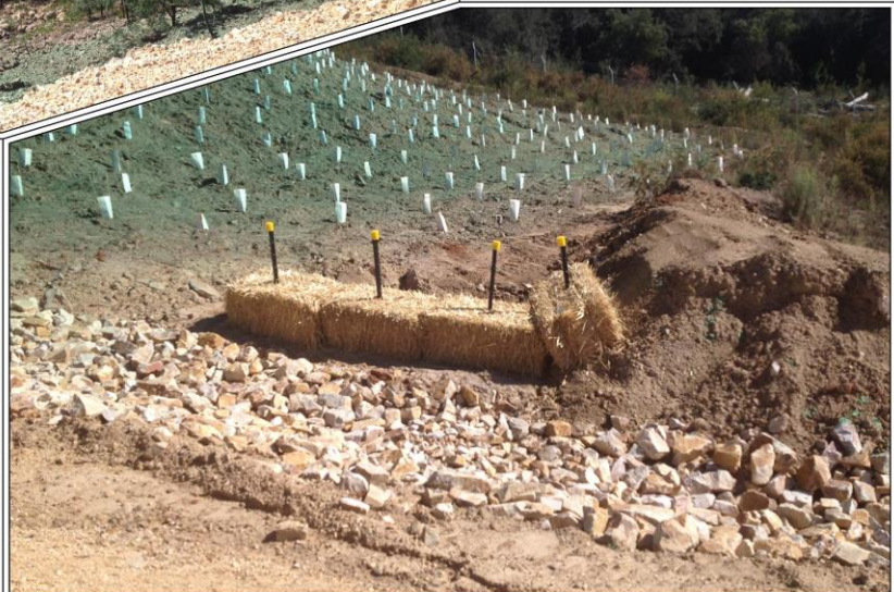
Plate 4: Tube stock and hydroseed batter of the Amenity Bund and Erosion Controls (Ref: IMG_3583)
