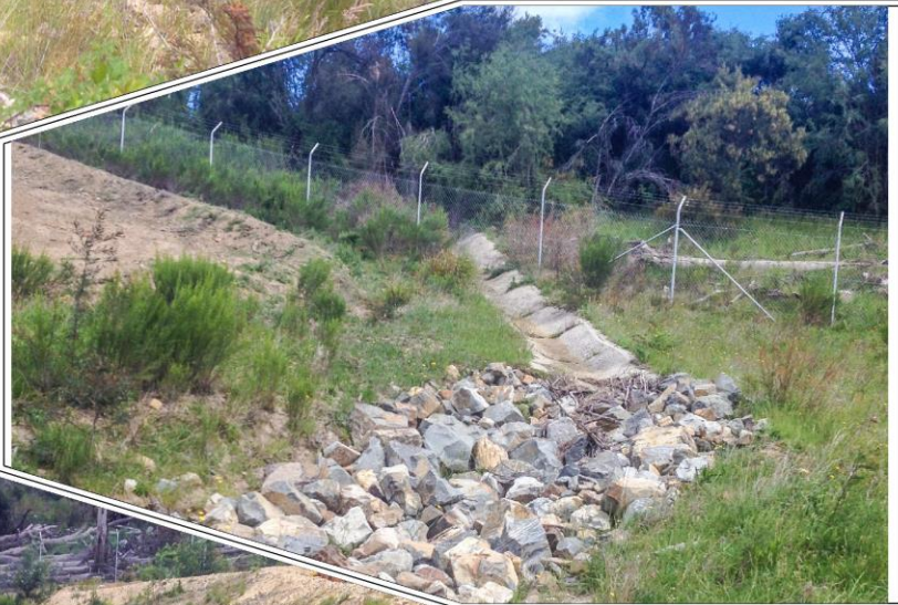
Plate 2: Concrete Drain from Great Western Highway Surface Runoff (Ref: D141116_IMG_1901)
