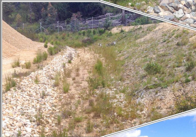
Plate 3: Open Channel from Northern Quarry Site Catchment (Ref: D141116_IMG_1904)
