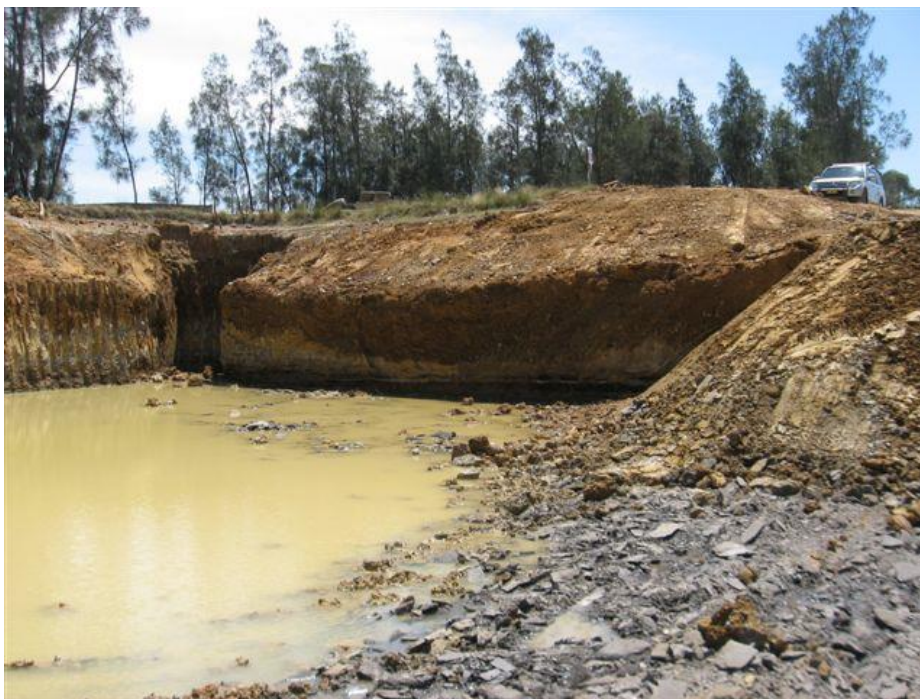
Sediment Pond 3 being de-silted
