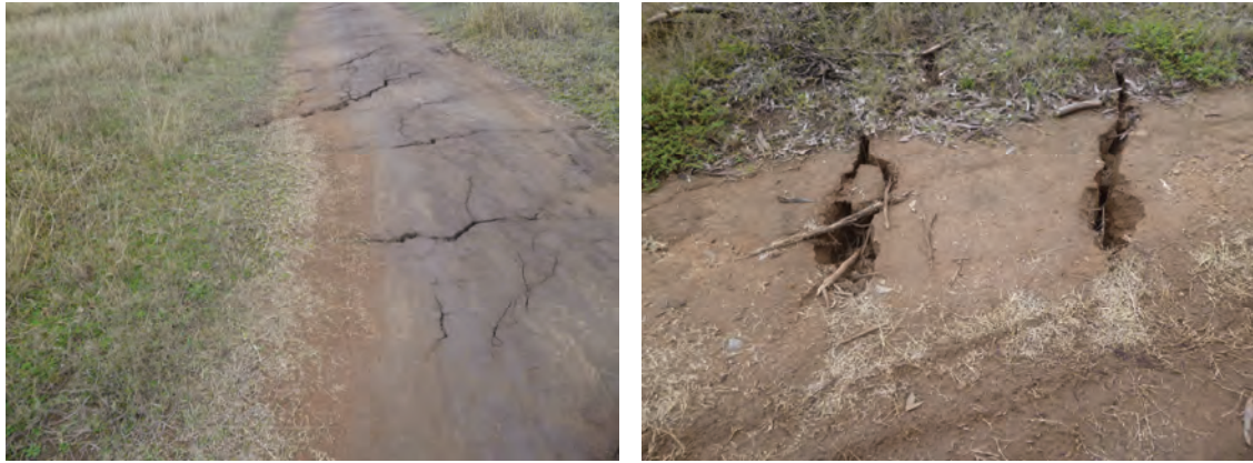
Fig. 4.6 Surface Cracking along an Unsealed Road above WYLW11
