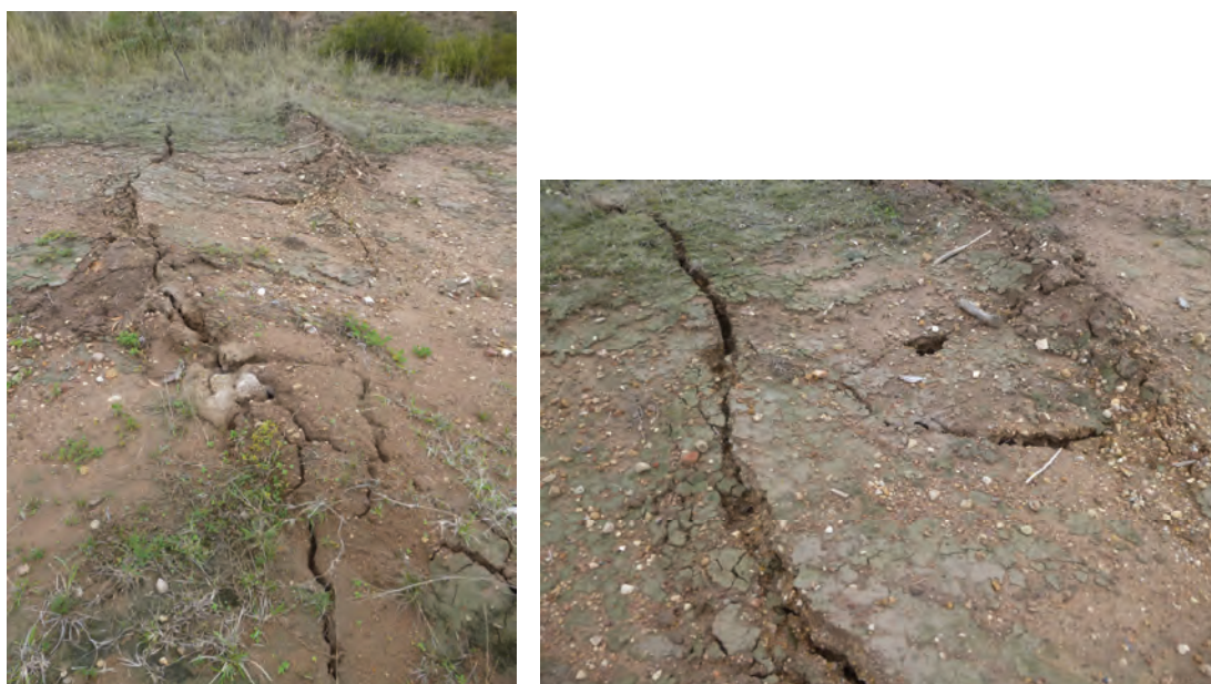
Fig. 4.5 Compression heaving along the North Wambo Creek Diversion due to WYLW11
