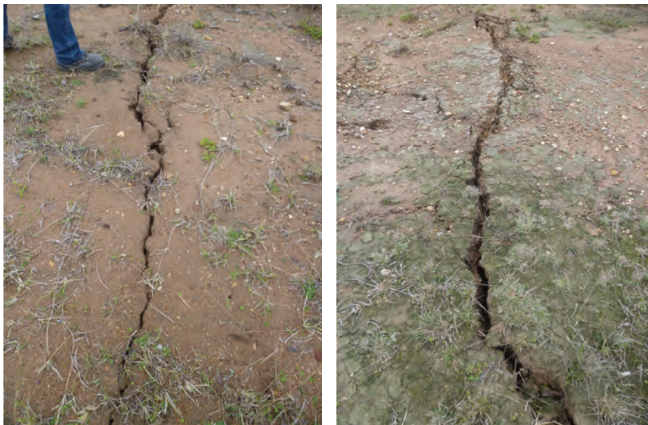
Fig. 4.4 Surface cracking along the North Wambo Creek Diversion due to WYLW11
