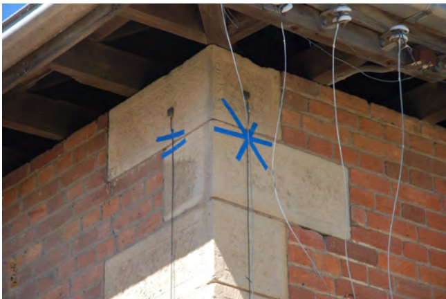
Figure 8: Attachment to top north-eastern corner of Building 'C'.
