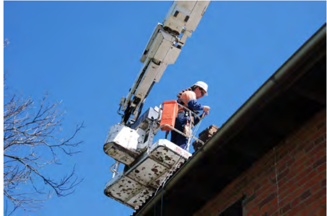
Figure 7: Accelerometers being attached to chimney of Building 'C'.
