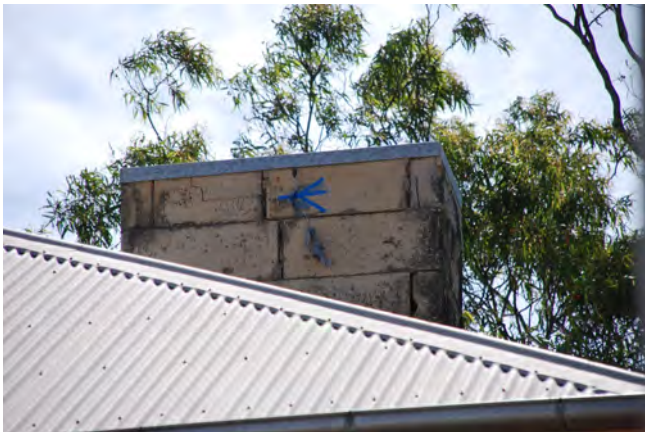
Figure 6: Accelerometer placed at top of southern chimney of Building 'A'.
