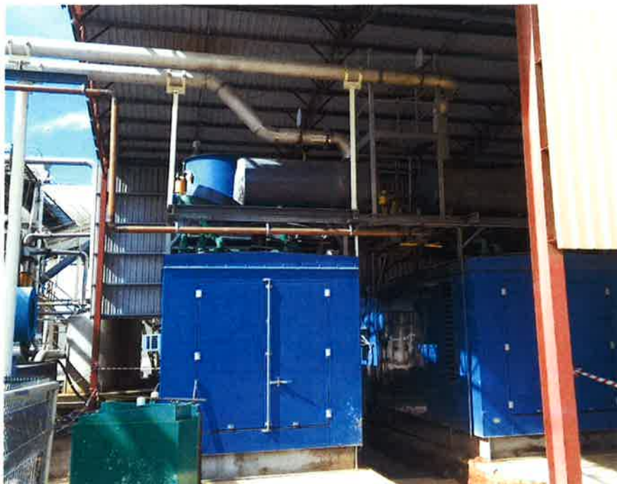
Figure 4: Cogeneration units contained within a soundproof enclosure
