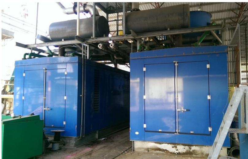
Plate 3: Generator's Steel Enclosures, Steel Awning area and Exhaust Mufflers
