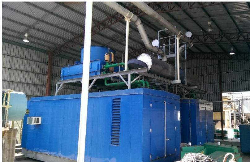
Plate 2: Generator's Steel Enclosures and Steel Awning area
