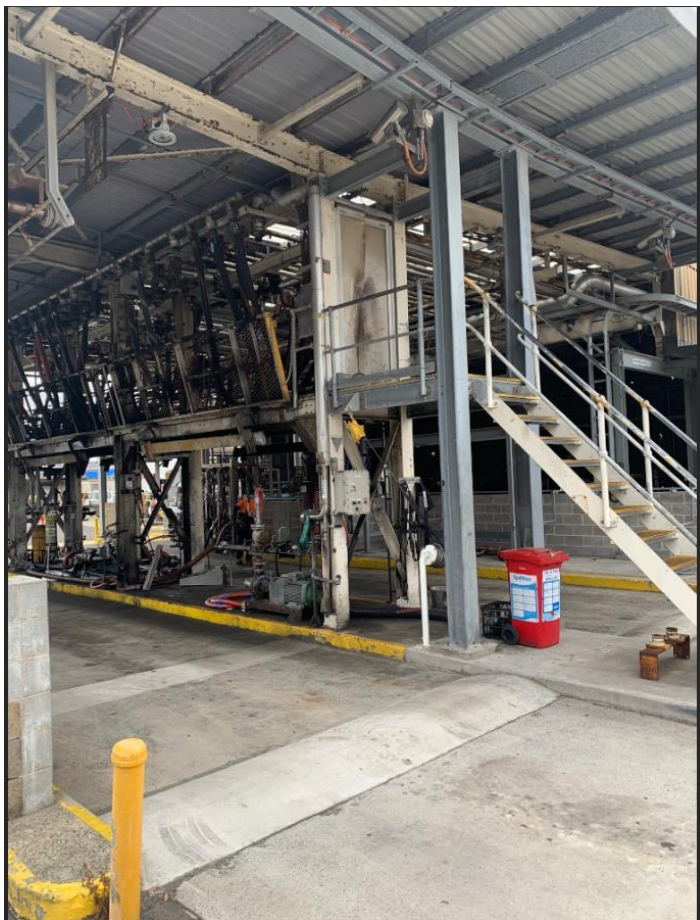
Gantry Bay 2 – rollover kerb to stop rainwater entering. Roof extension also visible at top right
