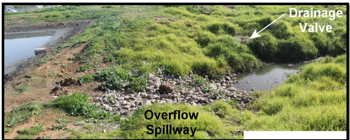
Figure 8: First flush pond to the left, overflow spillway and downstream channel and drainage valve (Source: Claus Environmental Engineering, 2014)
