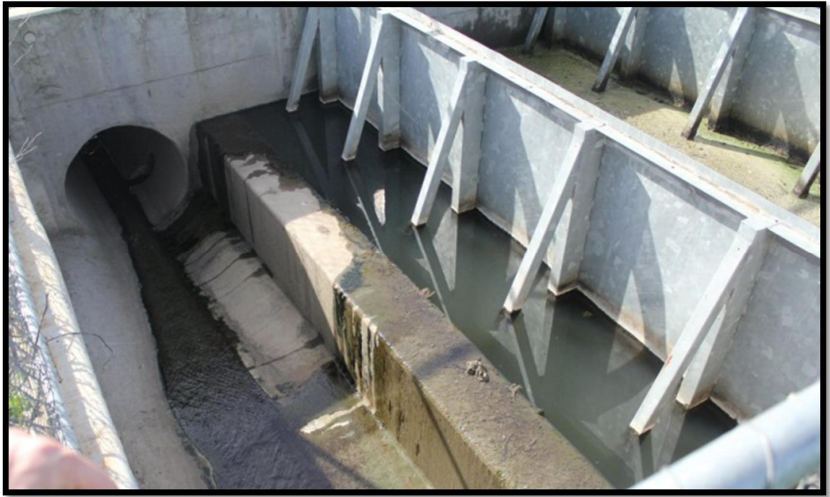
Figure 6: Final chamber of the baffle basin (Source: Claus Environmental Engineering, 2014)
