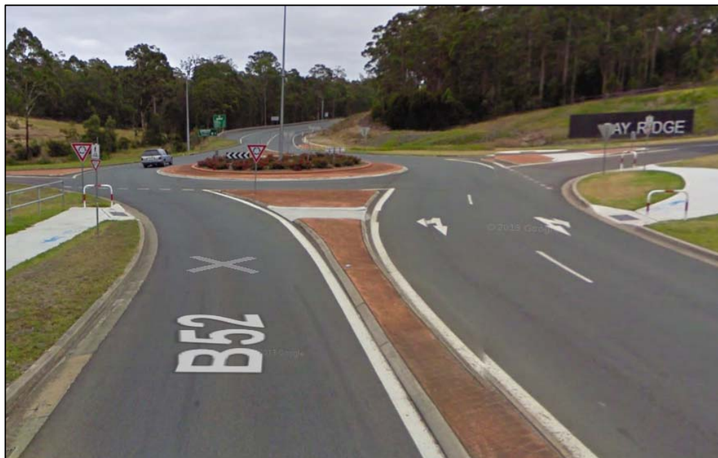
Figure 6 Princes Highway south of the site (looking north)
