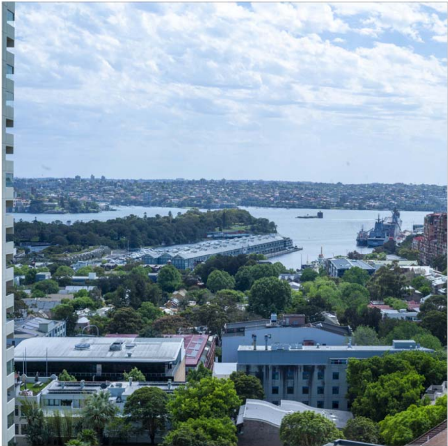
1. EXISTING VIEW - Standing
