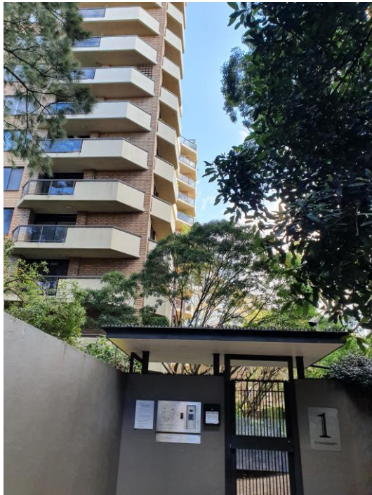
1 Tewkesbury Avenue, showing glazed balconies
