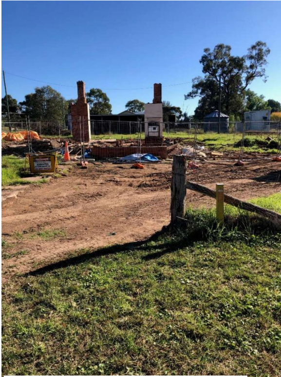
Figure 6: Site of demolished house, Wollar
