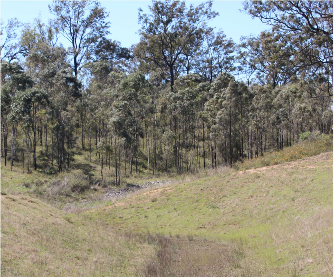
Eastern clean water diversion, 3 to 4m deep and travels up a steep slope.
